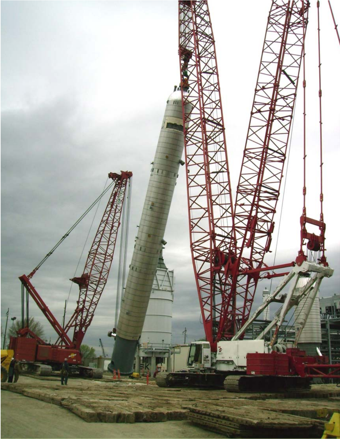
500,000 lbs Reactor Installation at the Holly Oil Refinery – April 2008
